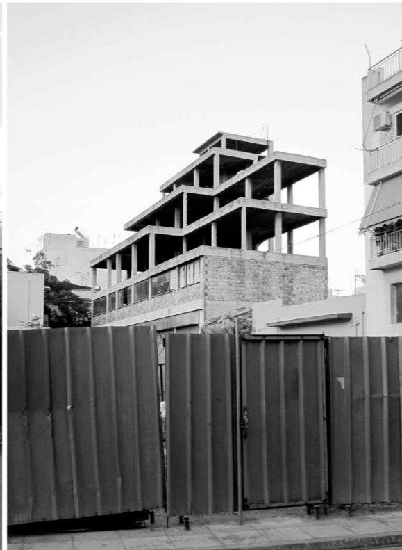
morphological typology: Upper level [UN] structure : multiple story / free standing / stepped floors municipality: Athens address: Paramithias 16 & Salaminos
